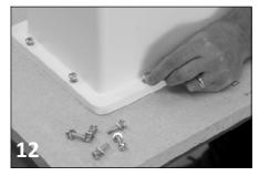
Re-position the sink and dry fit all the bolts to make sure everything is lined up correctly with the brass plugs.
