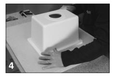
Position the sink over the cut-out on the underside of the worktop looking through the waste hole for reference. Check that the overhang is equal all the way round the sink.
