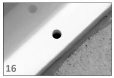
Gently place the sink into position making sure the holes in the sink flange sit directly over the brass plugs. Visually check that you have a continuous bead of adhesive around the sink flange on both sides.
