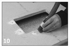
Once all the necessary plug holes have been drilled, make sure that the holes are free from debris and dust so that the brass threaded plugs are not impeded when fitting.
