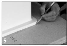
Once in position, mark small positioning points around the outside edge of the sink flange and onto the underside of the worktop so that you can re-position the sink accurately when moved.
