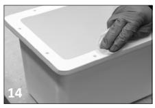
Repeat this process on the sink flange and leave both surfaces to air dry. To prevent any joint contamination after cleaning, be sure not to touch either of the jointing surfaces.
