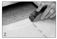
Key the underside of the worktop where the sink flange will sit using P240 grit paper lightly sanding round each side of the cutout. Ensure to remove any batch number print that may contaminate the adhesive.
