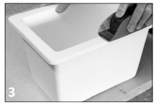
Using the same process, key all sides of the sink flange. Be careful not to sand the internal edge of the sink. Once complete wipe down both jointing surfaces using isopropyl alcohol wipes.
