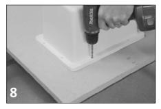
Re-position the sink to the underside of the worktop and carefully drill through the flange holes into the underside of the worktop to mark the hole positions using the same 6.5mm drill bit.
