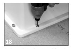
Continue to tighten the bolts until the spring washers have been flattened. After approximately 60 minutes (subject to room temperature) the adhesive will be cured and the worktop can be turned over to its face side.
