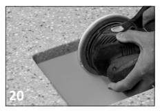
Using P240 and then P320 sanding discs and random orbital sander with extraction, sand away any residual adhesive until the worktop edge is flush with the sink and the joint is smooth.
