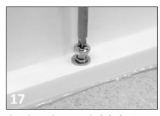
Place the washers onto the bolts (spring washer first) and insert the bolts through the flange holes into the brass plugs.
