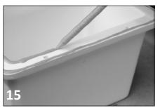
Apply a bead of worktop colour-matched adhesive to the entire inner and outer edges of the sink flange. You will have approximately 10 minutes working time (subject to room temperature).
