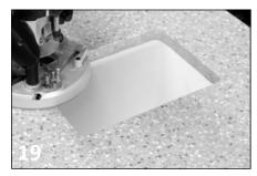
Using a router and a flush sink profile cutter, remove the excess adhesive and worktop overhang. Make sure you set the cutter to the correct depth (We recommend a test cut on a waste piece of material first).
