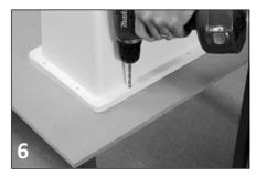
Remove the sink and place it on a waste piece of board making sure the sink is fully supported. Drill through the centre of the sink flange and into the waste piece of board using a 6.5mm drill bit.
